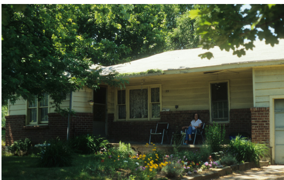
Wood frame, single-story bungalow style dwelling. Later expanded with a garage extension. Home faced with brick.
