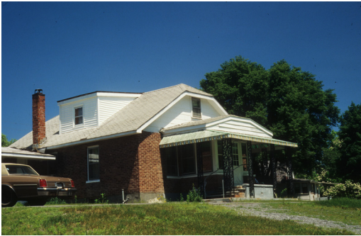
Brick and wood frame, single story bungalow style dwelling
