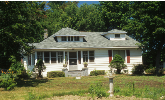
Wood frame, single story bungalow style dwelling
