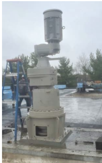
Figure 7-1: Mixer Drive Mechanism
