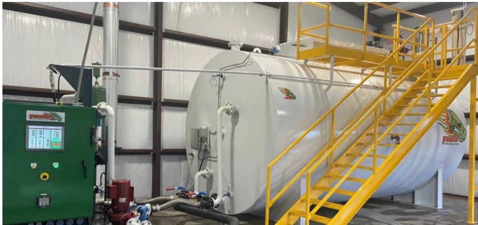
Figure 5-1: Example FOG Separation System Installation
