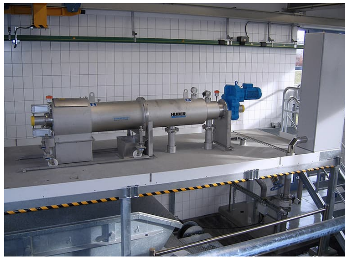
Figure 6-1: Strain Press Example Installation
