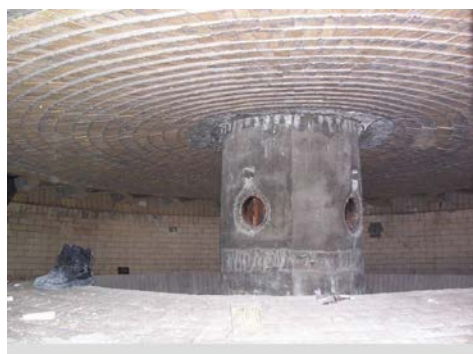
Refractory and Castings (portion of North done in 2024 as emergency)
