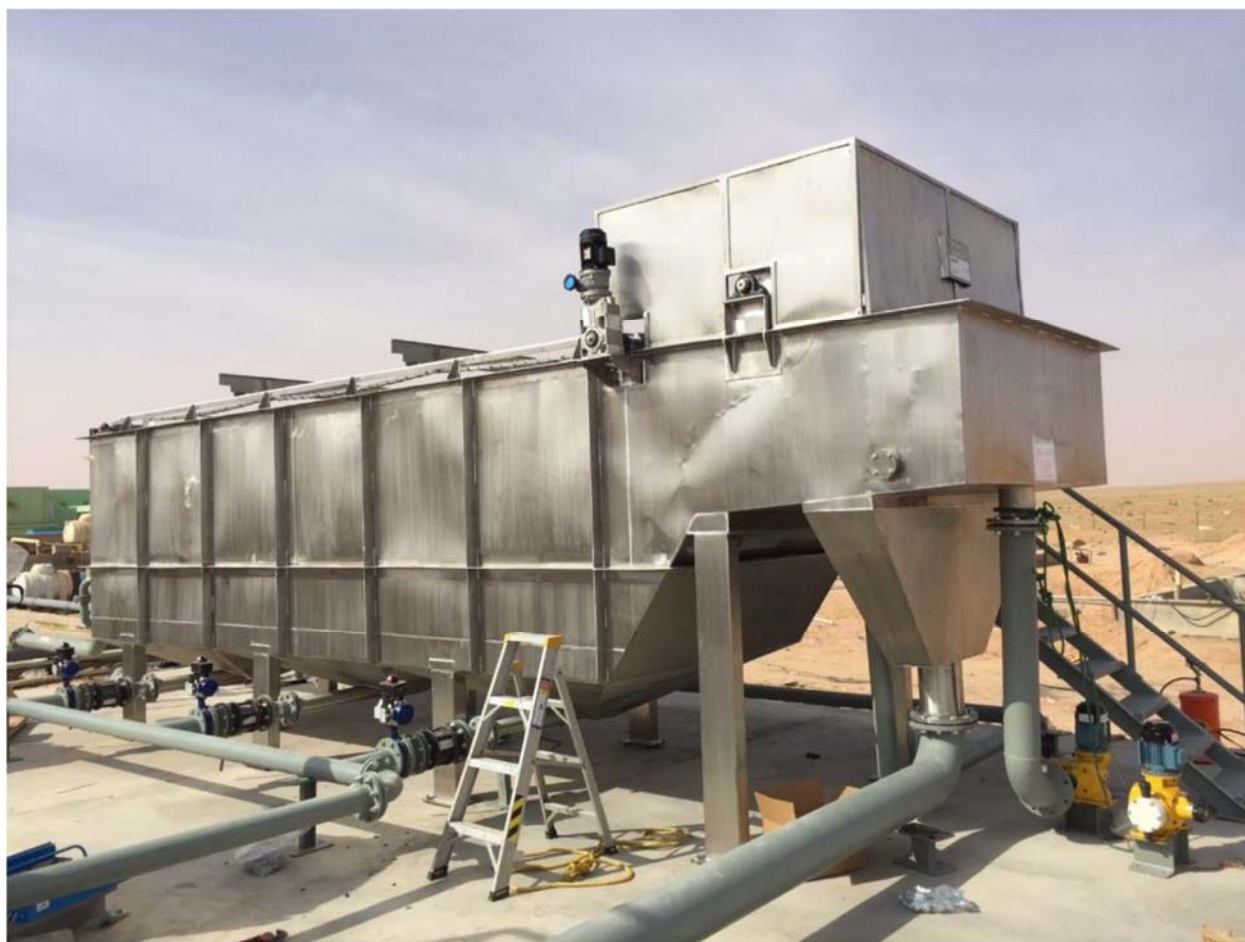
Figure 4: DAF (Typical)
