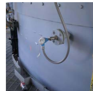
Thermocouple
