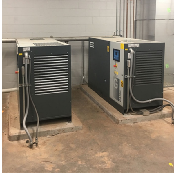
Compressors can be located indoors for weather protection and ease of maintenance
