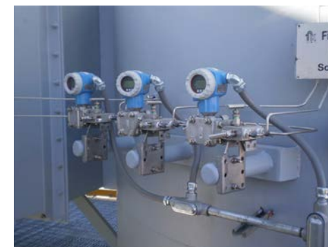
Differential Pressure Meters
