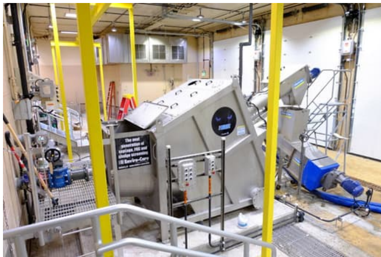
Figure 5-2: Example FOG Screen Installation
