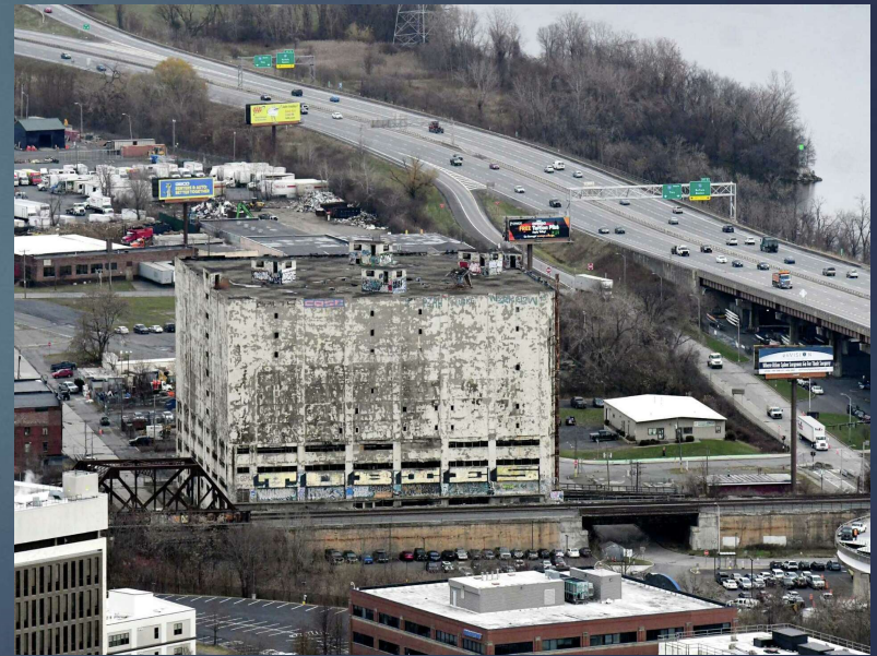
Albany Central Warehouse
