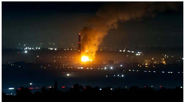
Moss Landing battery storage facility fire on January 16, 2025
