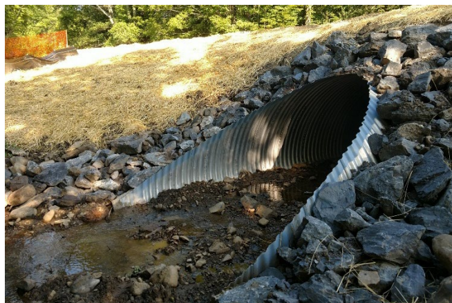
Replacement of Four Large Culverts Various Locations, Albany County
