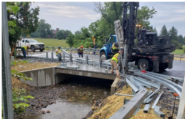
Construction Inspection Services for CR106 Culvert Town of Coeymans, Albany County
