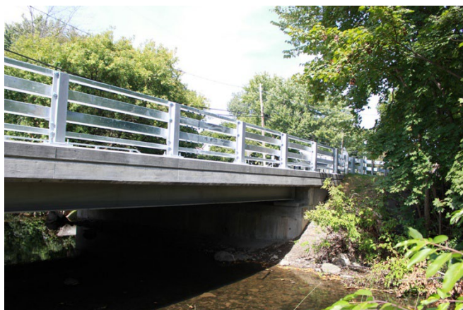
CR202 over Black Creek Superstructure Replacement Guilderland Center, Albany County
