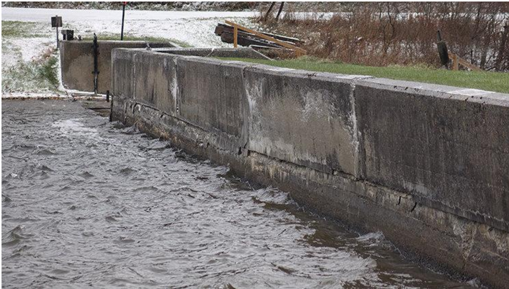
Helderberg Lake Dam
