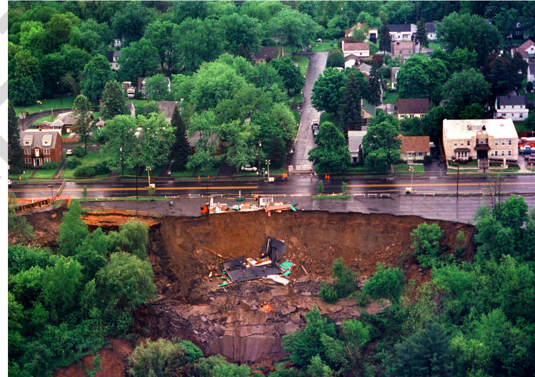
2021 Landslide in Delmar, NY (Source: Times Union)
