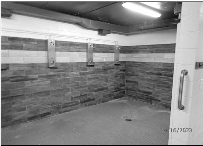
Locker room showers
