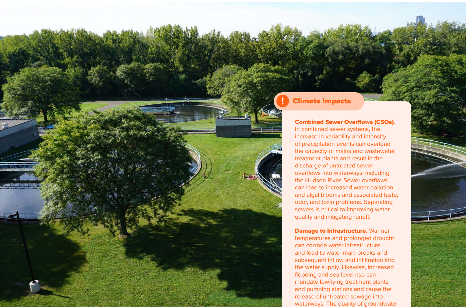
⌘ Albany County North Wastewater Treatment Plant Menands
