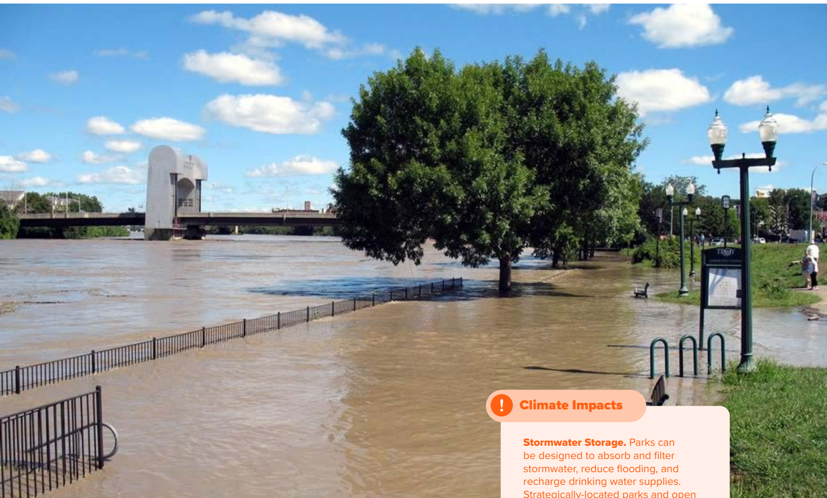
⚡ Hudson River Flooding, Troy, NY Hurricane Irene, September 2011
