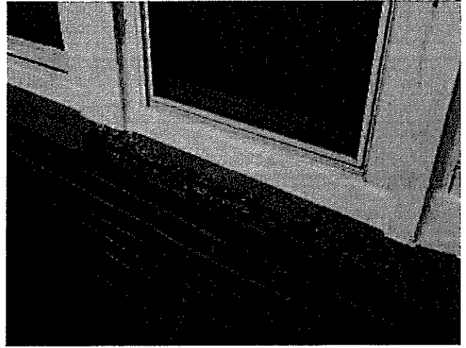
A-3 PRE-CAST CONCRETE SILLS
